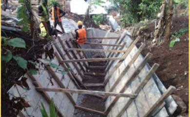
Formwork and reinforced concrete pouring by section
