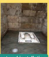
Models 1 and 2: installation of the urine separator seat and installation of the cabin cleaning wastewater collection system
