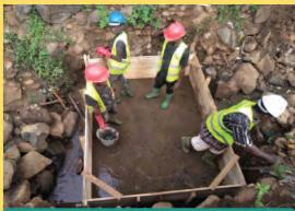
Formwork for casting the assembly anchoring mass on site 1
