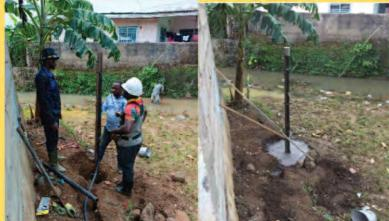
Installation of a pressure transducer central unit and view of the connection cable to the submerged module
