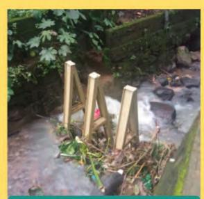
View of the completed 3assembly logjam trap at site 2 (after a rain)
