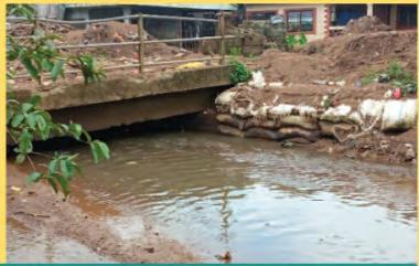
View of impacted earthbags after heavy rains, without being washed away by the flood.
