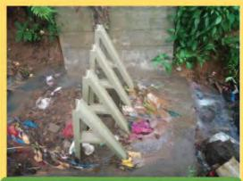
View of the completed 4-joint logjam trap on site 1
